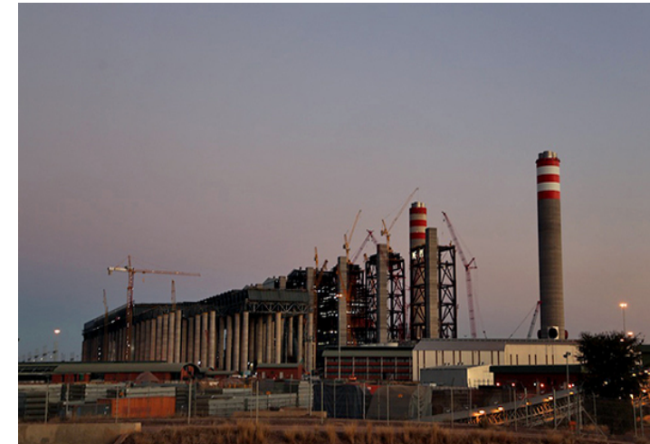
Medupi power station
