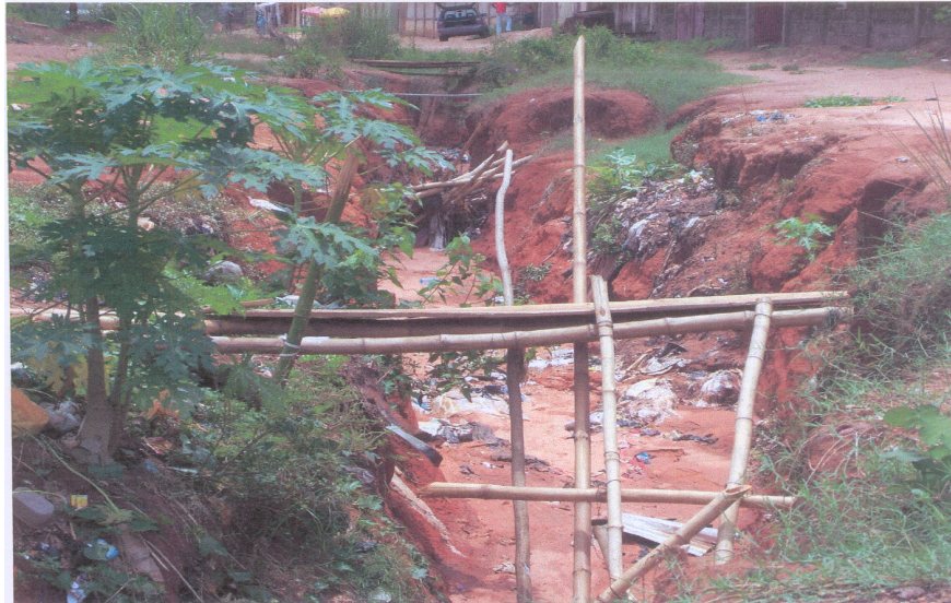
Fig. 4: Abandoned Building destroyed by flood, in Umuna Orlu, Imo State
