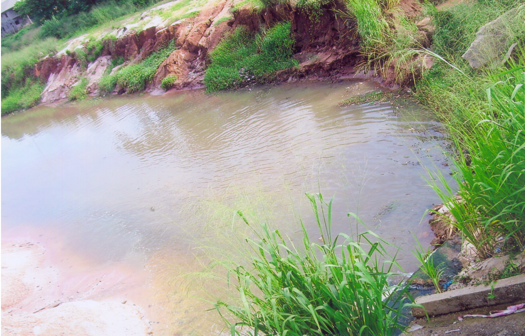
Fig. 2: Ikenegbu road in Owerri, Imo State destroyed by gully erosion
