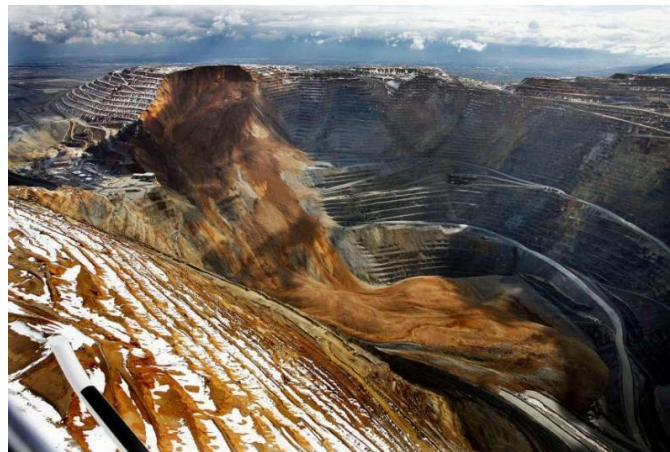
Figure 1. Slope failure at the open cast mine.
