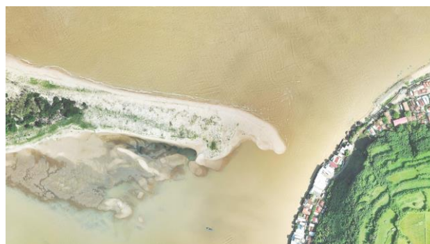
Figure 2. Tien Chau tidal inlet captured by drone in 2019. It is observed that many houses are constructed at the down-drift barrier of the inlet. The sandspit at the updrift side moving toward the Southside.
