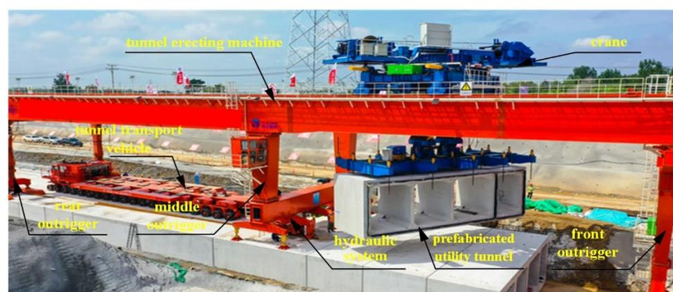
**Figure 1.** Tunnel erecting machine of prefabricated utility tunnel.
