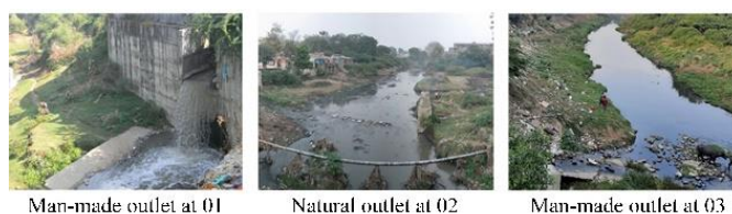
Figure 15. Sewage/storm water outlets.
