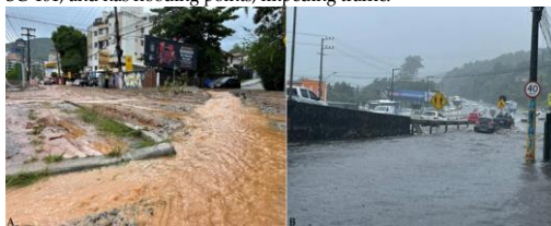
Figure 4: Damages caused from rainfall. Source: G1 Santa Catarina.
