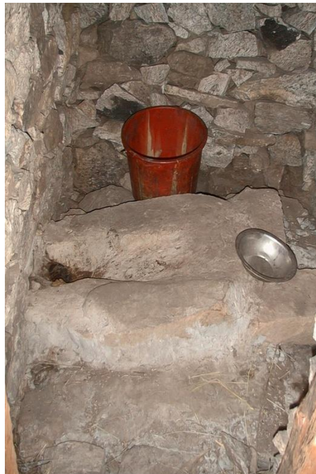
Figure 3. The interior of a typical latrine. Note empty flush bucket.
