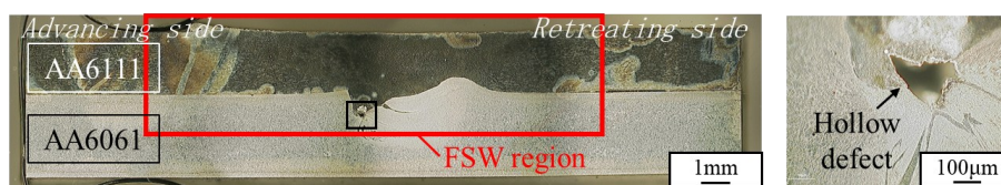
(a) Cross-sectional image. (b) Hollow defect. Figure 3. Cross section of defective FSW joint.
