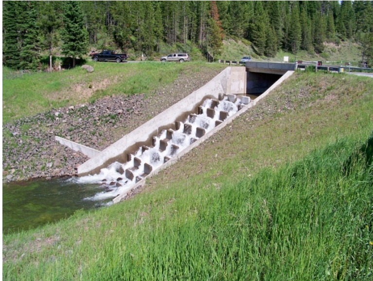
48 Figure 1. Example baffled chute spillway in Bozeman, Montana USA (photo from C. Brown).
