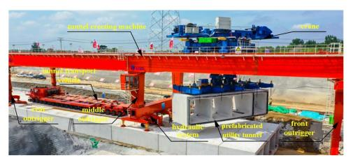
Figure 1. Tunnel erecting machine of prefabricated utility tunnel.
