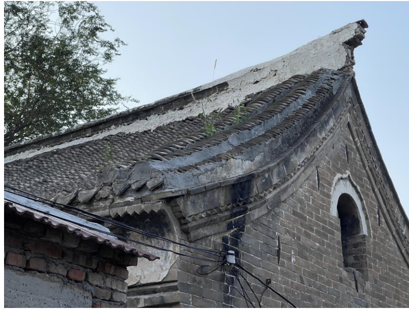
Figure 1. The rivets in the gable wall area work with the beams and columns to secure the architectural ceiling.
