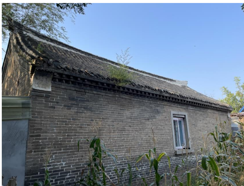
Figure 4. Repair works to the walls.
