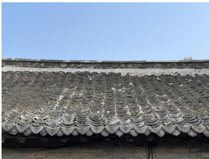
Figure 3. Roofing and tile processes and techniques.
