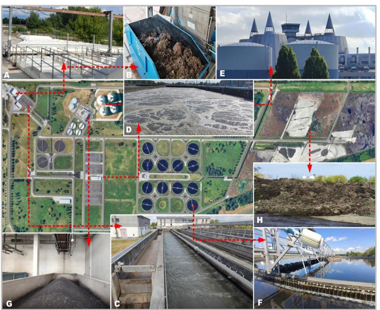
The central wastewater treatment plant of the City of Zagreb, Croatia, showing: (A) inlet channel and pumping station, (B) screening facility for removal of primary impurities, (C) sand and grease trap, (D) aeration basin for biological wastewater treatment, (E) facility for mesophilic anaerobic digestion of sludge and cogeneration plant, (F) secondary sedimentation basin, (G) facility for dehydration and conditioning of digested sludge, and (H) disposal site for treated sludge.
