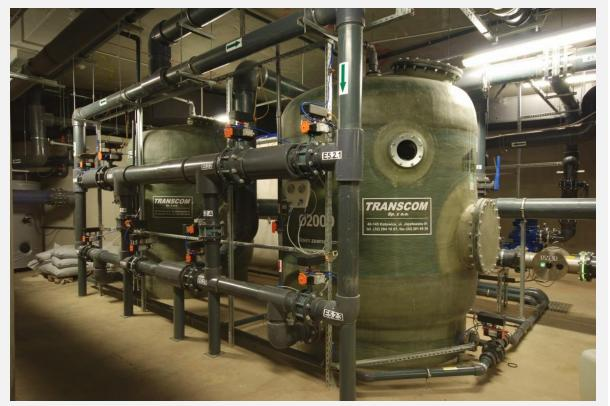
Fig. 1. The multilayer pressure filters
