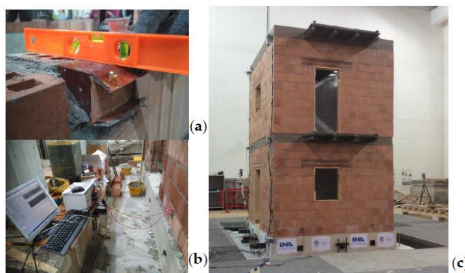
Figure 3. Full-scale tests: (a) placement of the smart brick in the masonry; (b) setup for the electrical measurements; (c) picture of the tested building
