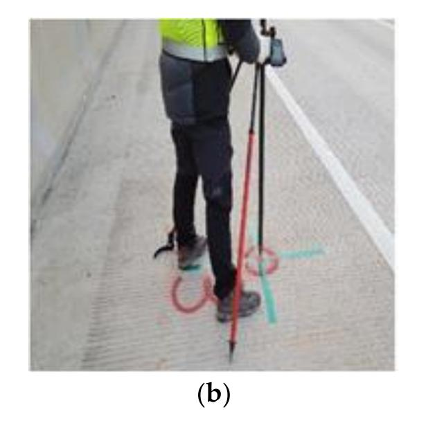
Figure 1. Wonjudaegyo Bridge, Korea: (a) Aerial view with control point locations; (b) Installation of control points before flying UAV.
