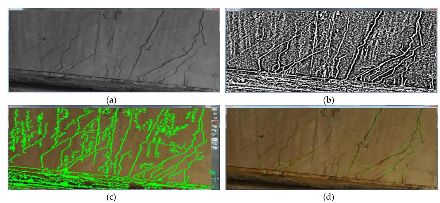
Figure 4. Results of crack detection in the Wonjudaegyo Bridge, Korea: (a) Data extracted from channel L (luminance); (b) cracks using Gaussian adaptive threshold method; (c) cracks after extracting area boundaries; (d) final cracks overlaid with image.
