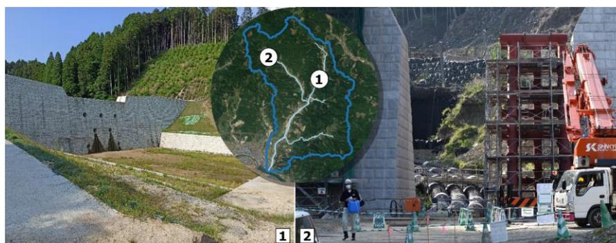
**Figure 7.** Illustration of the sabo dam constructed in the AK River. (a) closed-type sabo dam AK16, ©M. Dumont, 2022; (b) slit-dam type sabo dam OT15-6, ©V. Siccard, 2022.
