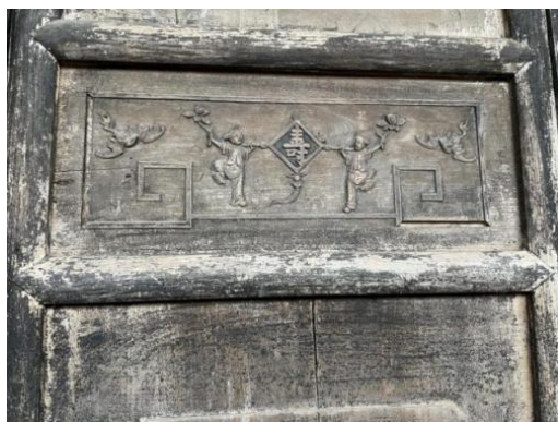
Figure 3. Carvings on the doors and windows of the Han Family Compound.
