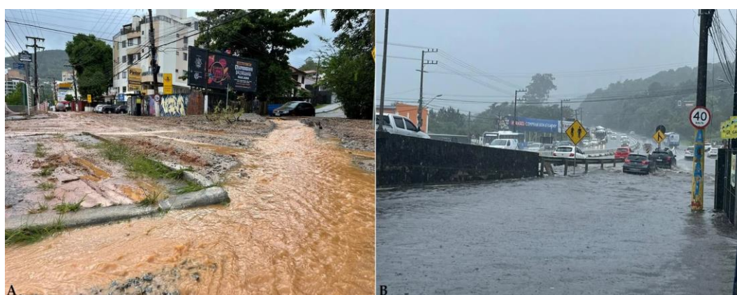
Figure 5. Damages caused from the December 2022 rainfall. Source: G1 Santa Catarina.
