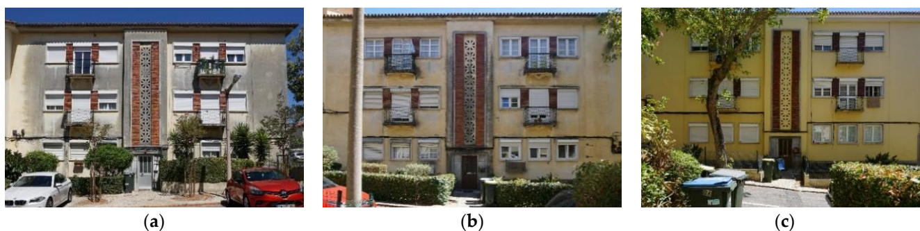
Figure 1. Façades' analyzed: (a) Buildings 4; (b) Buildings 7; (c) Buildings 9 (adapted from [1]).
