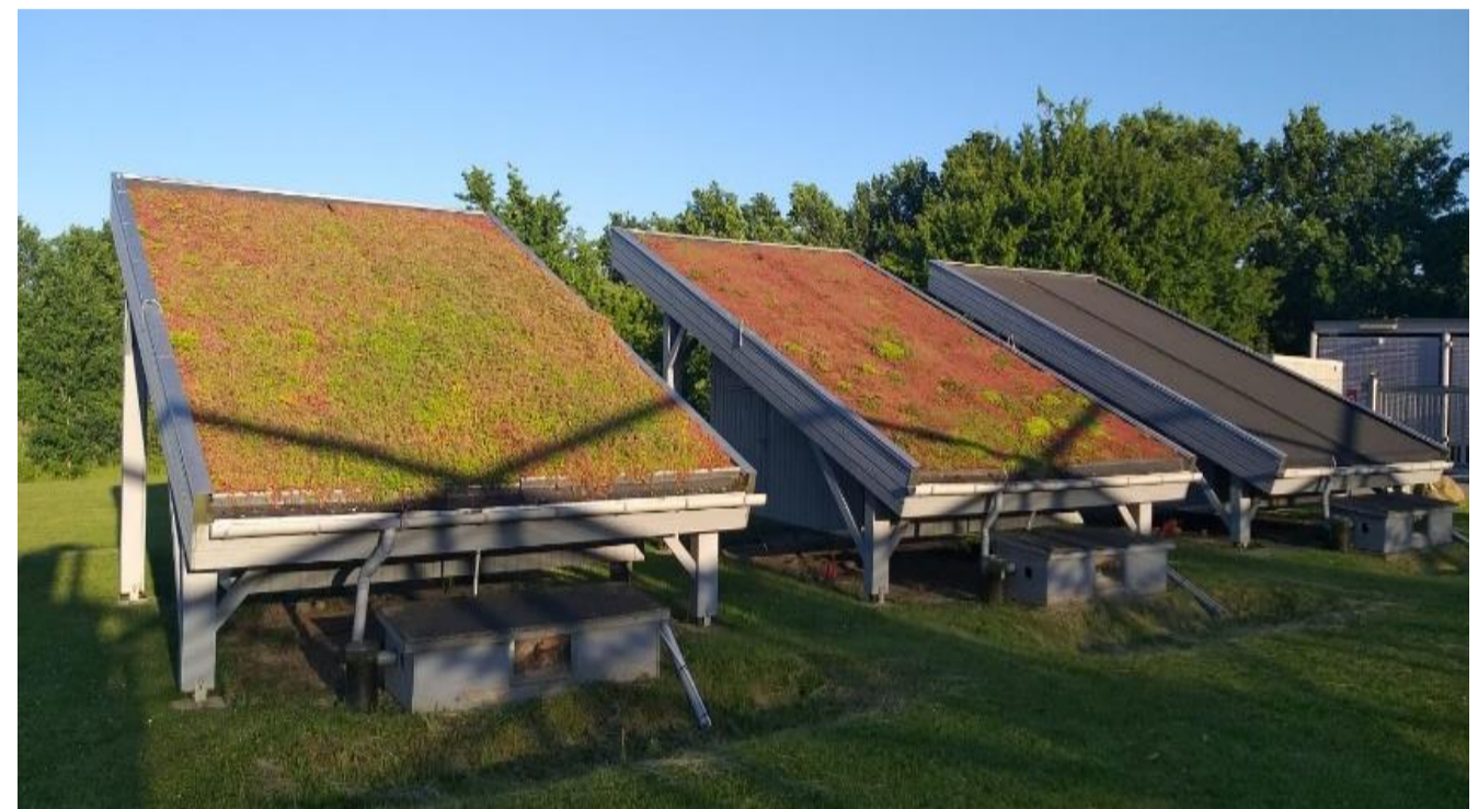
Green roof pilot system
