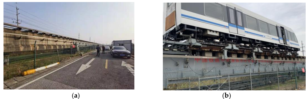
Figure 3. Pictures taken on the test site: (a) exemplary concrete beam; (b) test vehicle passing by a simply supported steel beam.
