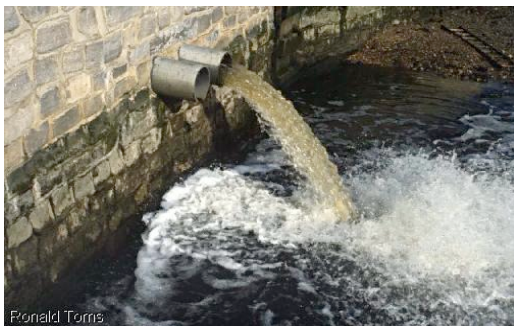
Point source discharge
