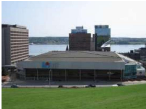
Halifax Metro Center (Canada): Making use of existing structural reserves to allow increased snow and equipment loads on the roof
