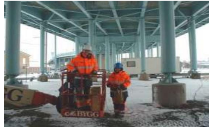
Göta Bridge (Sweden): safely extend the lifetime of the ageing bridge
