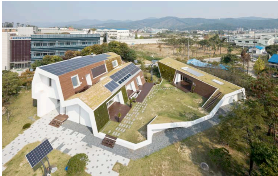
Figure 8. Aerial view of Kolon e+ Green Home. Well visible are the greened roof, facades, roof-integrated PV generators and solar thermal collectors. The Kolon headquarter building is visible in the background left.
