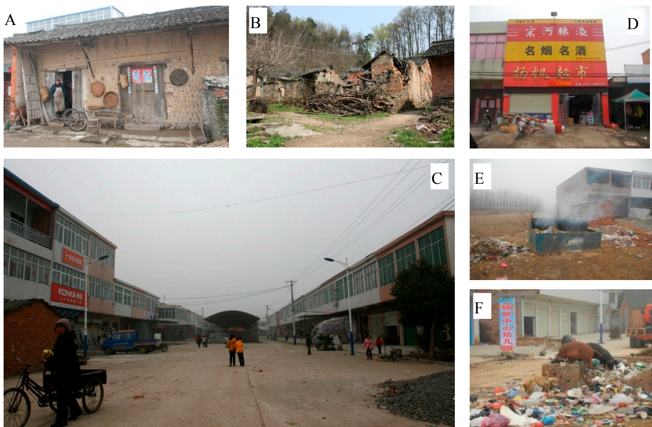
Figure 1. Jigsaw of Yang-Fan Village (A: vernacular mudbrick dwellings; B: abandoned housing in ruin; C: stereotyped modern houses and tasteless public space; D: store signs and advertising cause visual clutter; E: discarding and burning domestic garbage; F: livestock eating the discarded garbage on the street).
