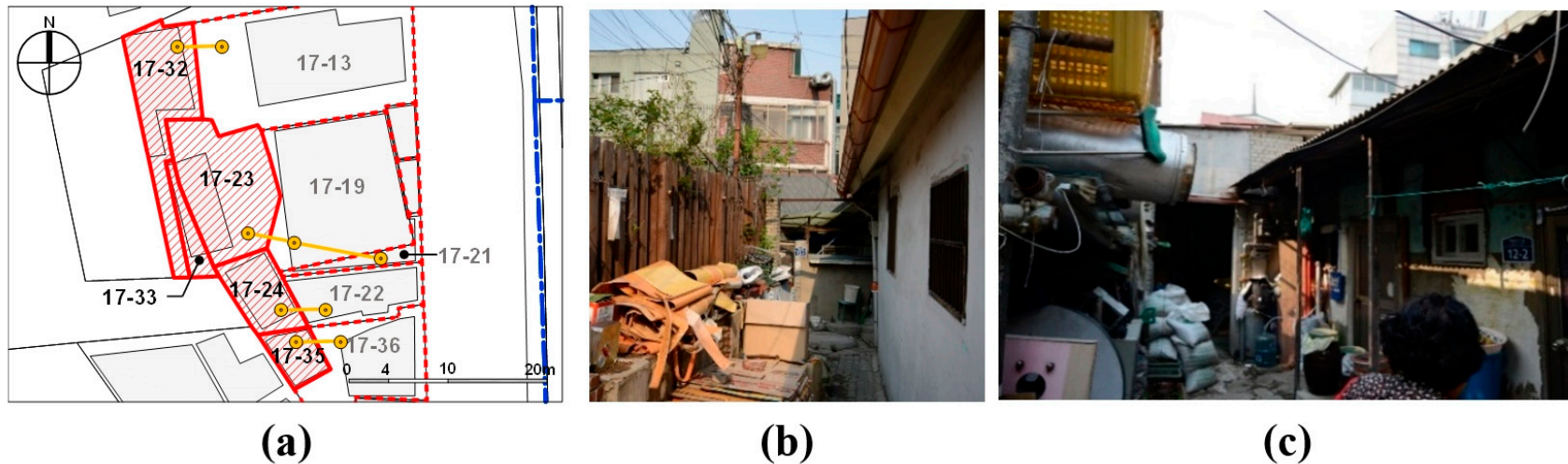
Figure 10. (a) Situation map around 17-32, 17-23, 17-33, 17-24 and 17-35 Changsin 3 dong. (b) (c) Field pictures of 17-32, 17-23, 17-33, 17-24 and 17-35 Changsin 3 dong
