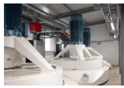
Figure 3. Flywheel Energy Storage
