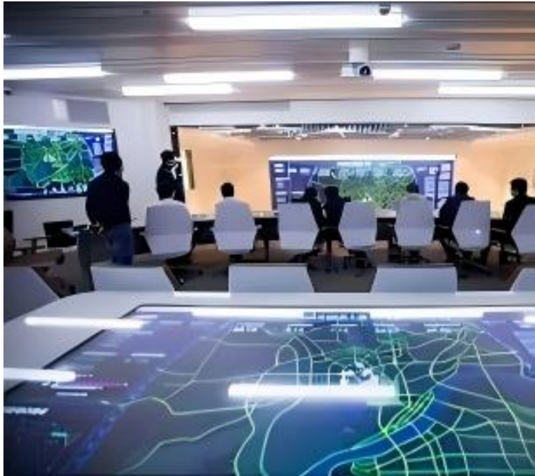
Figure 1. City Brain control-room environment in Hangzhou
