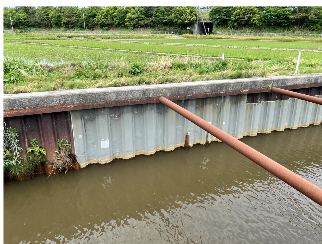
③ Ultra-thick polyurethane-resin coating system
