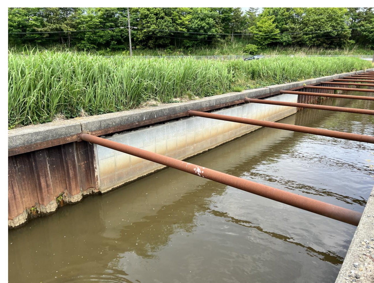
④ Precast concrete panel lining
