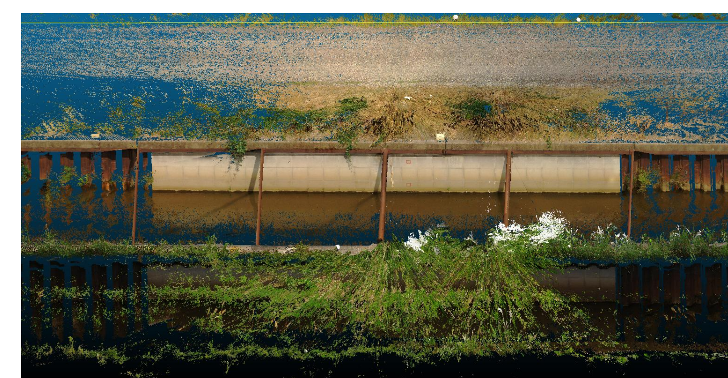
Precast concrete panel lining system
