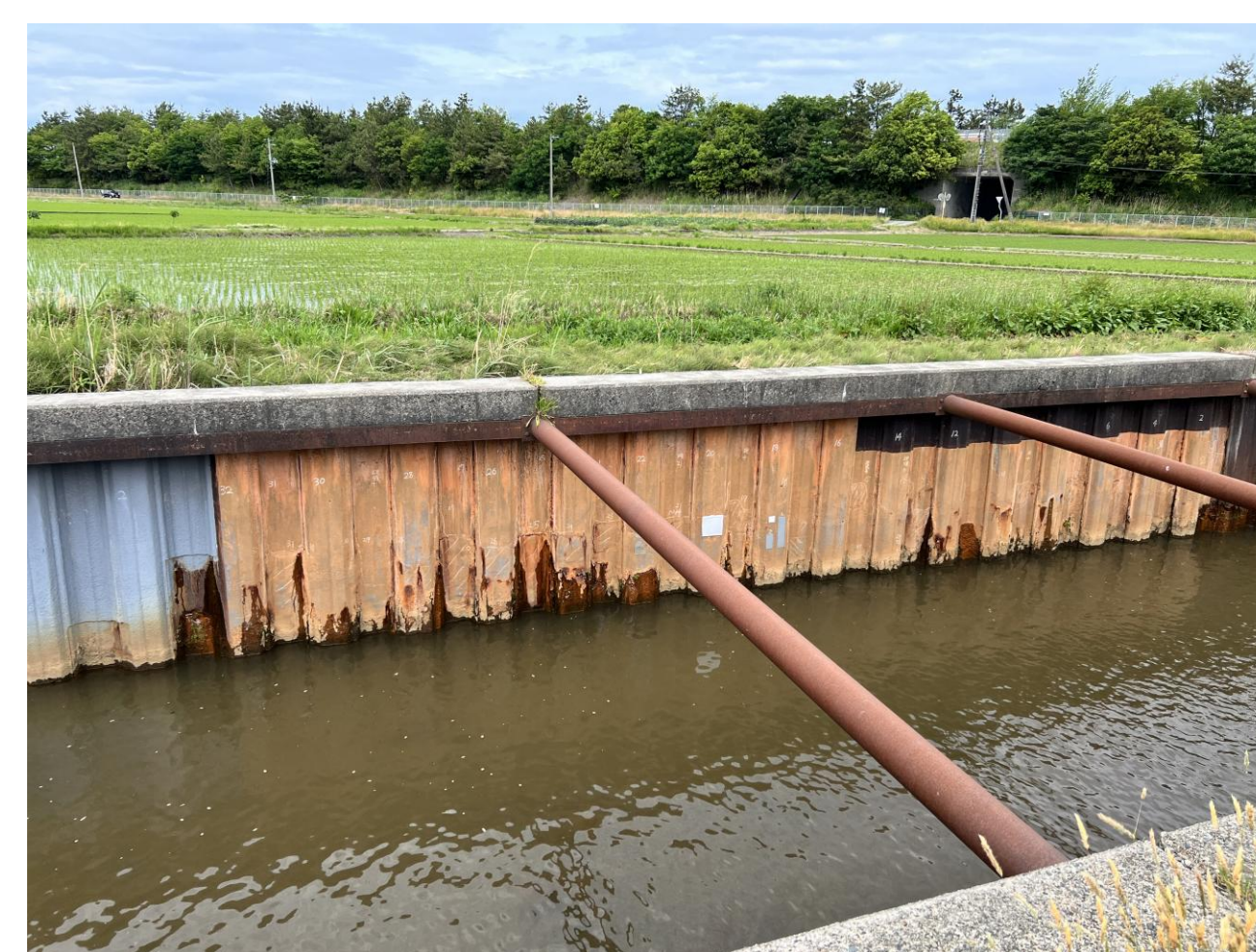
② Thin-film epoxy resin coating
