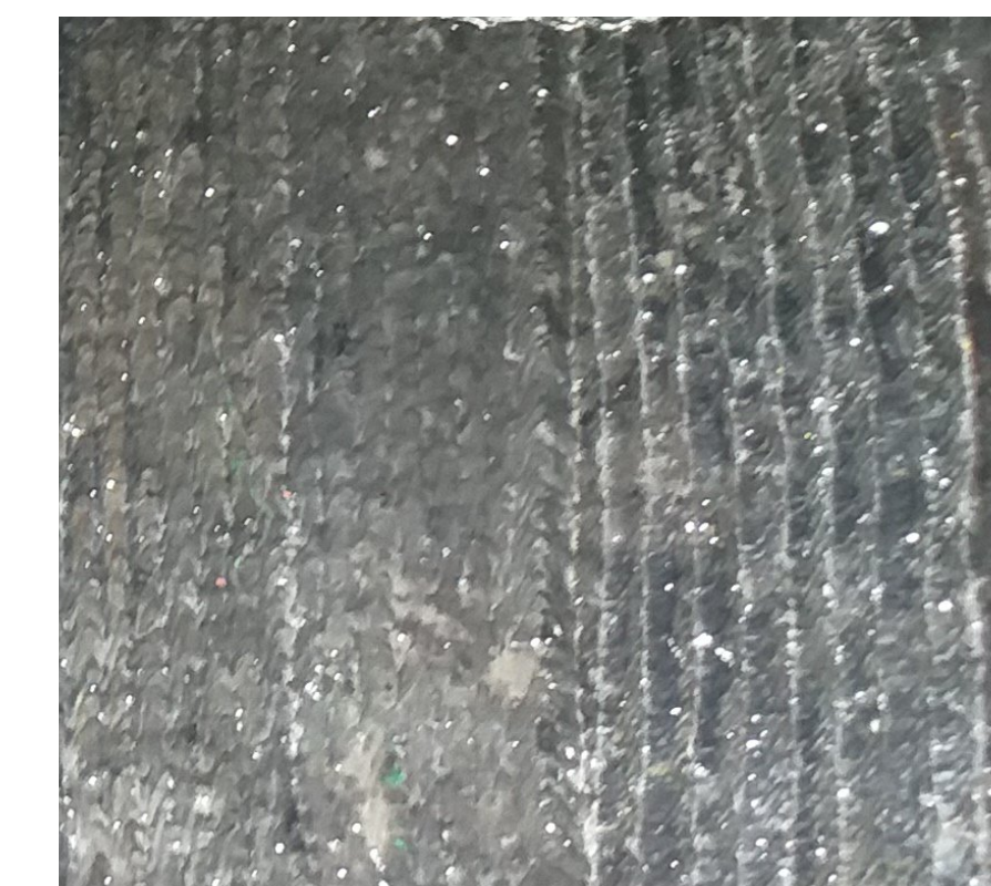
Figure 4 Restored surface of the pipe /without grinding/
