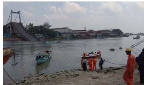
Figure 1. Myaungmya bridge after the collapse
