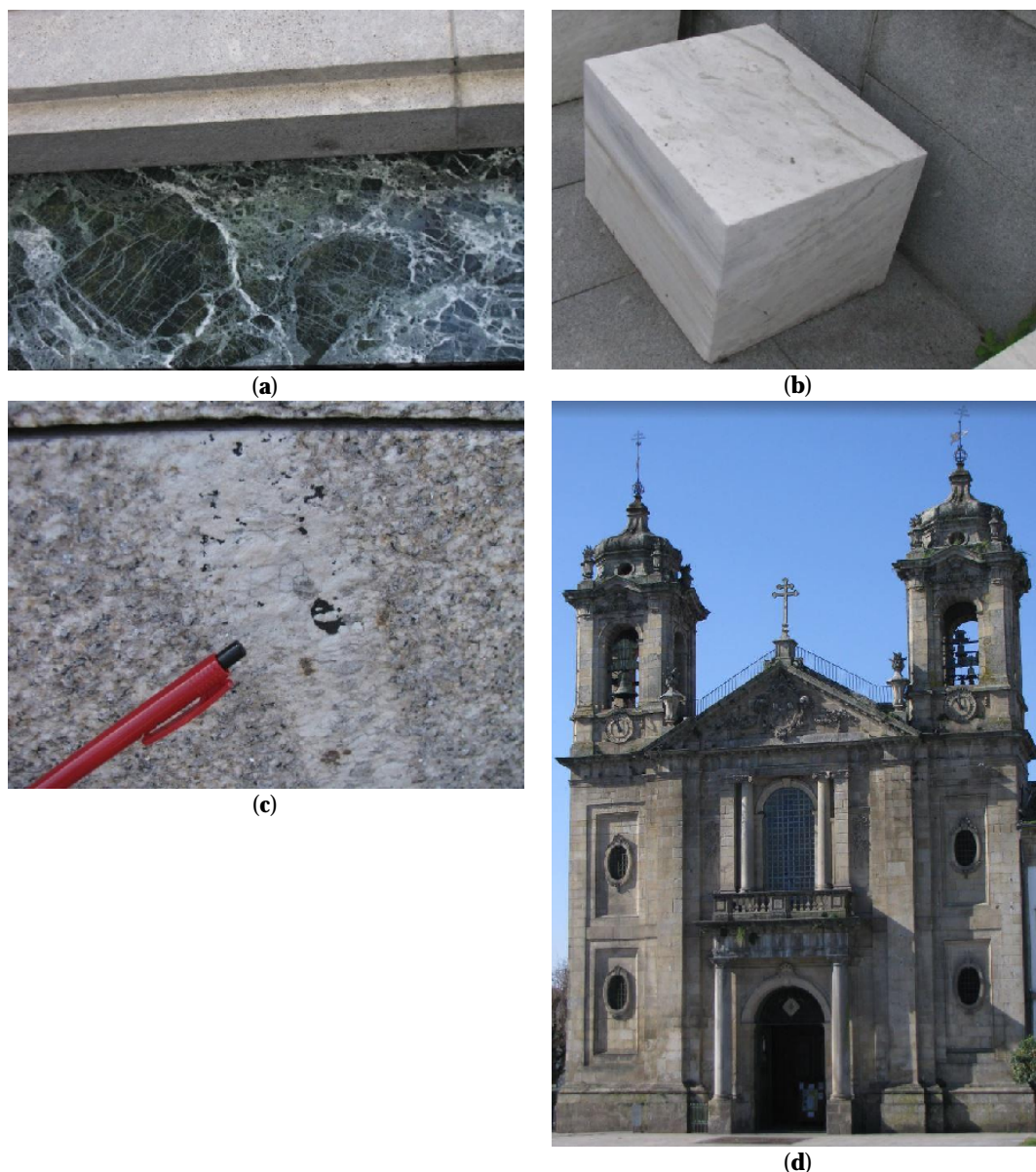
Figure 3. Stamps from built structures: (a) Juxtaposition of granite stones (similar to the local stone) and exotic green breccia; (b) marble block with planar structures that illustrate apparent variation of dip with view plan; (c) pegmatite veinlet on a granite stone; (d) image from the main façade of the Populo's church in Braga (Portugal).
