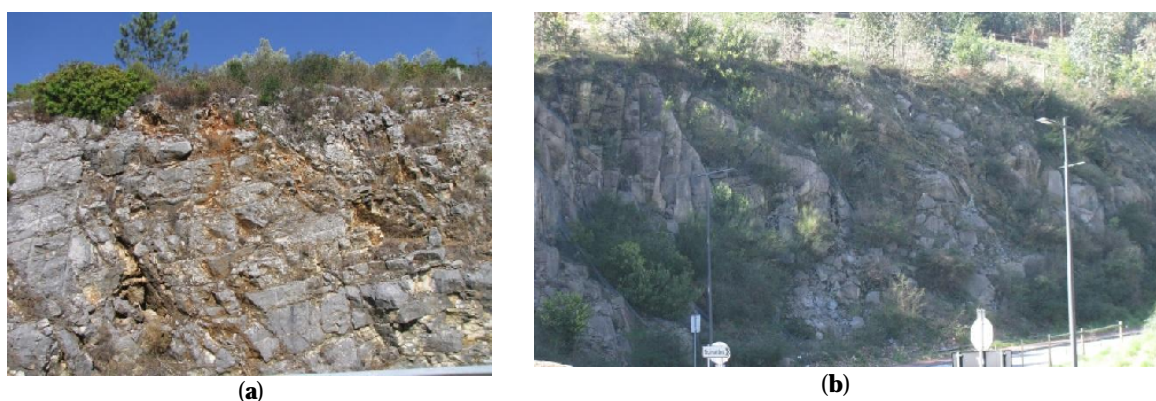
Figure 2. Stamps from anthropogenic rock-cuts: (a) road slope on a limestone mass showing bedding, joints and the effects of weathering (terra rosa); (b) road slope on a granite mass showing jointing that can promote rock movements, supporting net (to minimize that hazard) and natural recovery of vegetation.
