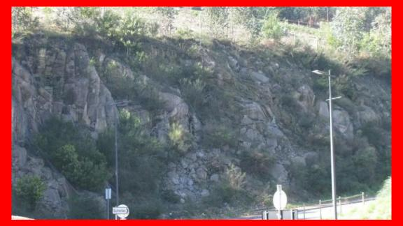
Presence of rock boulders within saprolite zones (relevant for discussions of geotechnical survey), characteristics of rock masses with relevance for geotechnical classifications, including joint length and joint walls coating (which can be related to mineralogical concepts), conditions for rock failure and intervention to minimize these hazards (metallic net).
