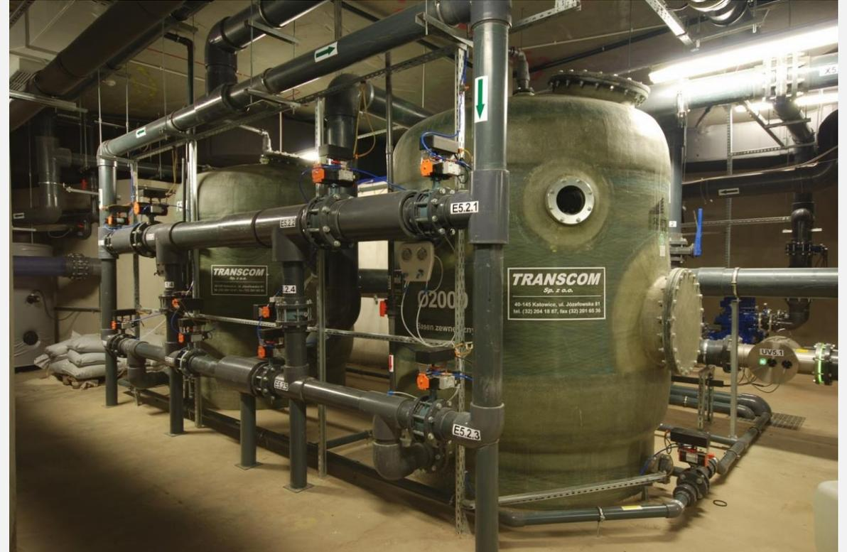
Fig. 1. The multilayer pressure filters
