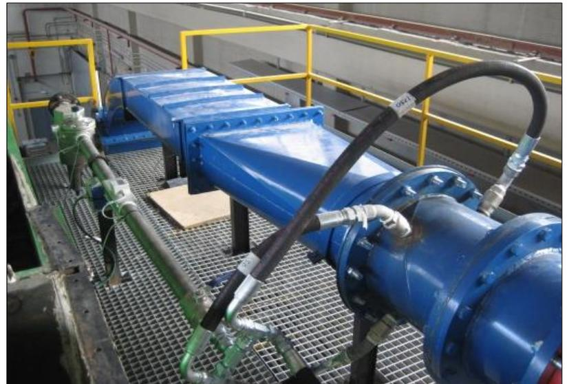
Figure 9. Air – water mixture box
