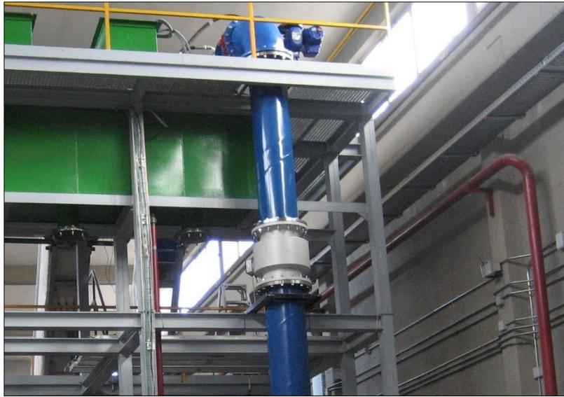
Figure 10. Water electromagnetic flowmeter
