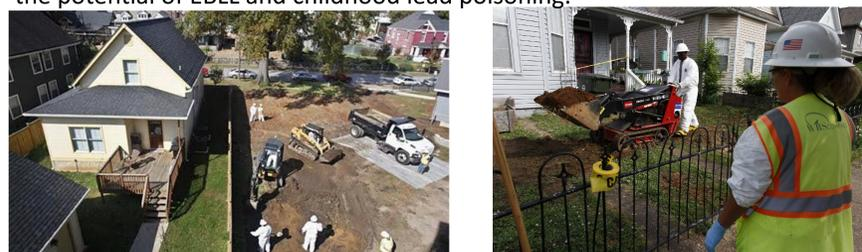
**Figure 2.** EPA workers replacing the contaminated soil of affected South Chattanooga properties.<sup>4</sup>
