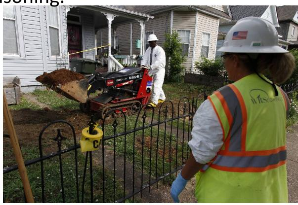
**Figure 2.** EPA workers replacing the contaminated soil of affected South Chattanooga properties.<sup>4</sup>
