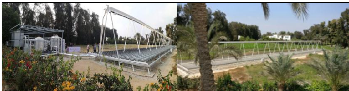
Figure 1. SEKEM LFR multi-generation plant.
