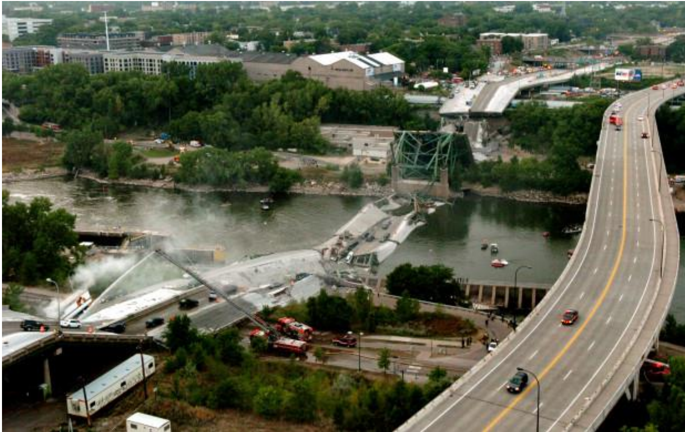
August 1st 2007, Minneapolis (Minnesota, USA): I-35W Mississippi bridge collapse killed 13 people
