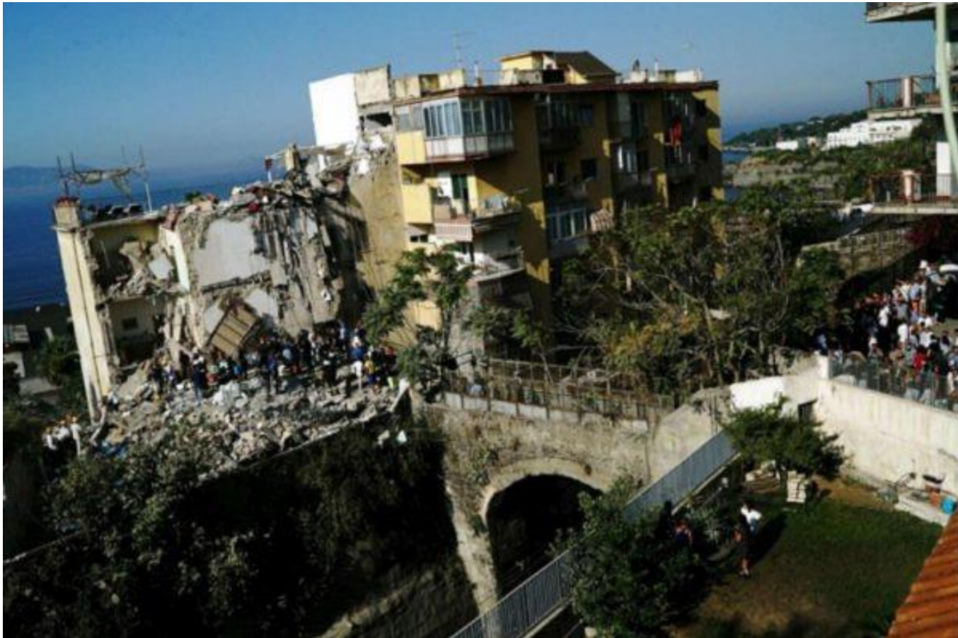
July 7th 2018, Torre Annunziata (Italy): residential building collapse killed 8 people
