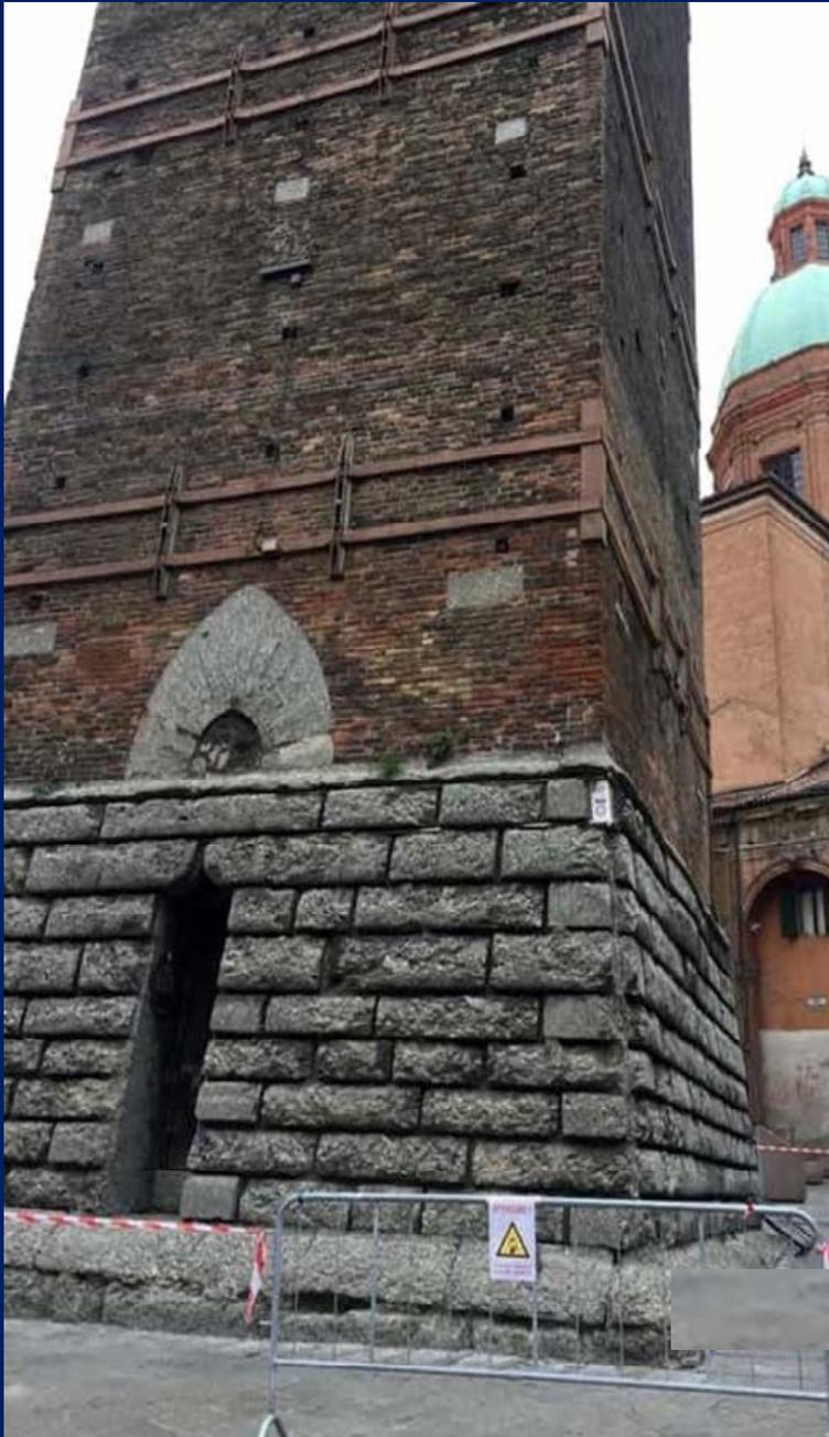
The Garisenda Tower, built around the same time, is much smaller (48 metres) but with a steeper leaning (3.22 m) due to an early and more marked subsidence of soil and foundation.
