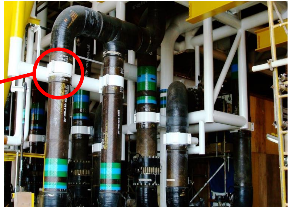
CEMENTED BELL & SPIGOT ADHESIVE JOINT
