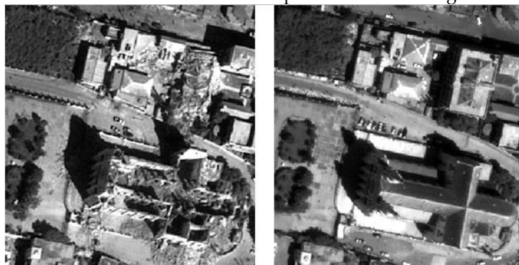
Figure 2. The right image is before the earthquake, and the left image is after the earthquake.
