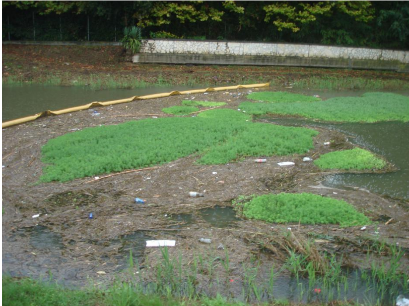
Lack of periodical cleaning during dry weather
