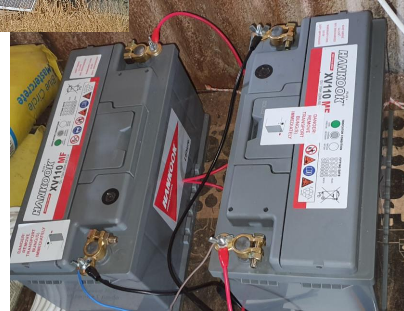
Figure 4. a, Top-left – siting of the two 150W solar panels facing due south, b, Bottom-right – two 110Ah lead acid batteries used to supply modules with power
